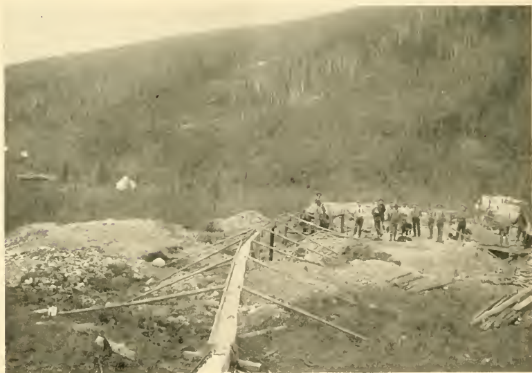
Claim No. 12, Eldorado Creek.—Mining by shafts sunk to bed rock, the dirt raised in buckets by windlasses, is dumped into a sluice box. Over $20,000 was taken from one of these 12 x 16 feet boxes.
